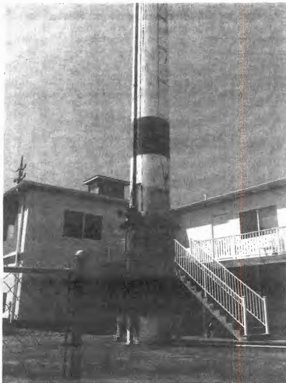
Figure 4: Exterior Elevator (Decommisioned)
