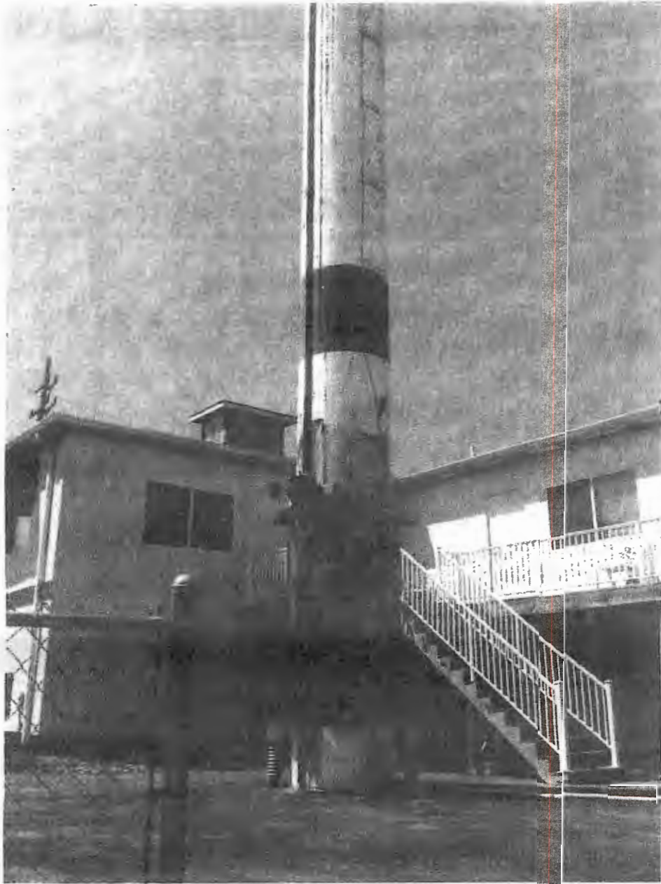
Figure 4: Exterior Elevator (Decommisioned)
