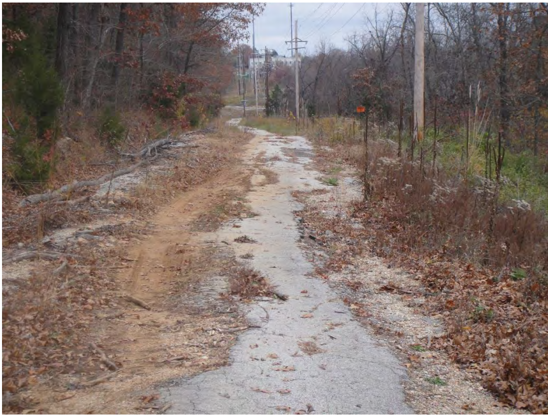
Photo looking east along Golf Rd. Same severe deterioration conditions evident. Note overhead utility line running length of road.
