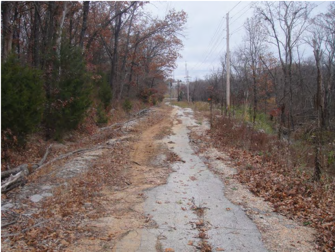
View looking east along Golf Road.
