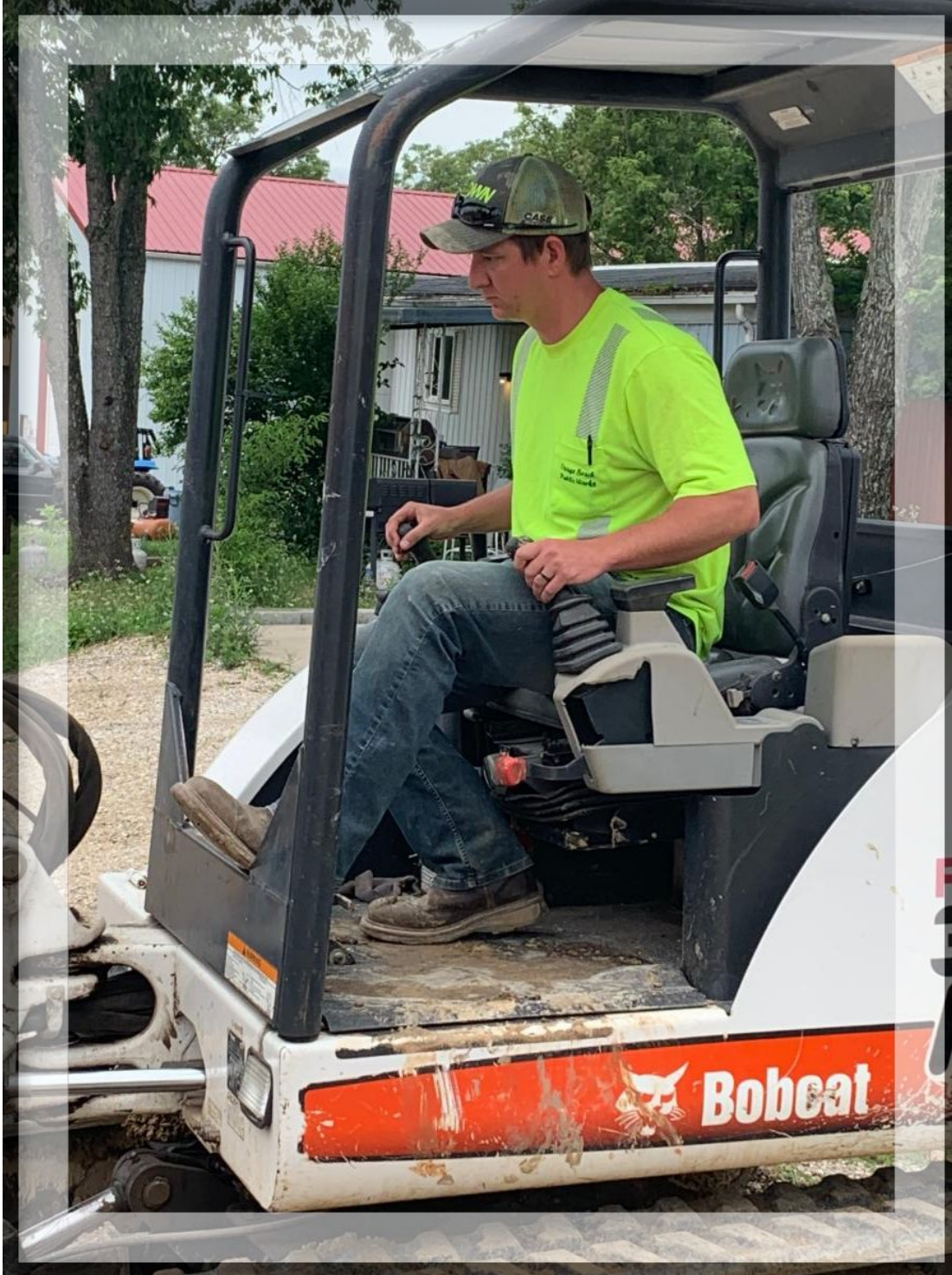
Public Works Water Department employee, Caleb DeVore, on a water project.
