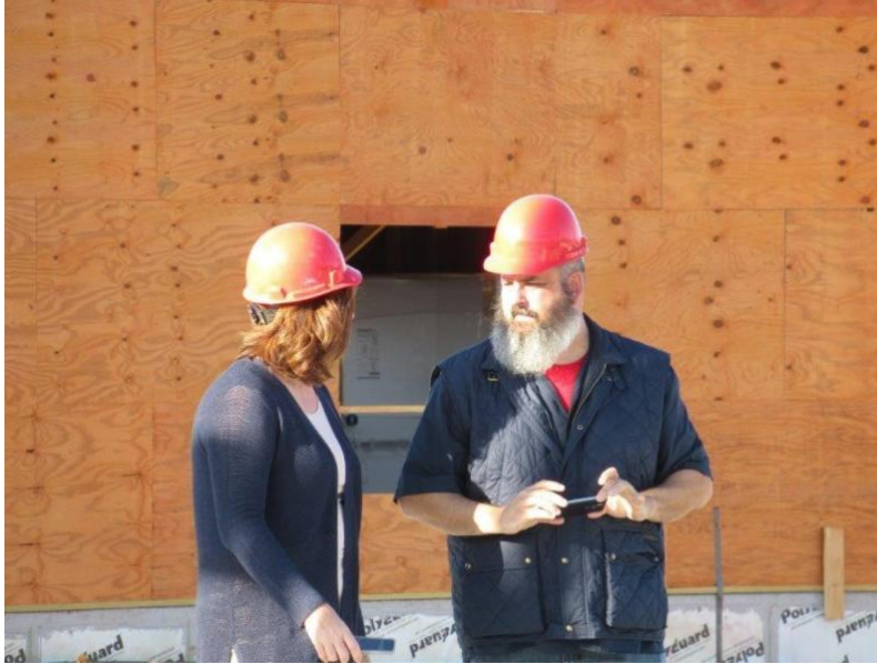
Ron White and Jeana Woods onsite at Arrowhead during construction.
